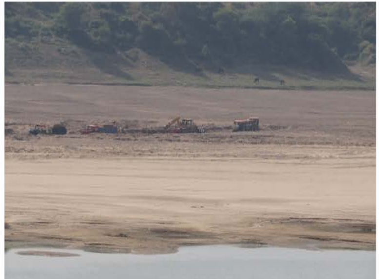
Figure 56. Sand mining at Tighra-Rithora turning, Madhya Pradesh side of Chambal River, using heavy industrial equipment for loading sand, such as "JCB" backhoes shown here. Sand is moved to high ground near the riverbank, and loaded on large lorries for long-distance transport to major construction sites. Such activity was evident at this site from Sept thru Dec 2016.
