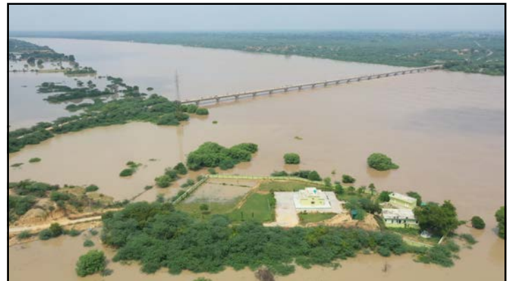
Fig. 102 Another view of the Sashon bridge during peak monsoon, showing the recently constructed UP Forest Department "rest house" complex entirely surrounded with high water, with the exception of a connecting roadway. Gharial utilize side channels and nullas as waterways to stay out of main flows.
