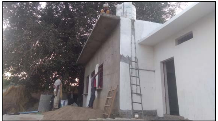
Fig. 108 Final construction phase involved painting the exterior and finishing windows and doors on the upstream base at Katrinapur. This facility now allows the GEP field team to live and work close to the Chambal at Baroli sandbanks, a traditional breeding and nesting site for resident gharials.
