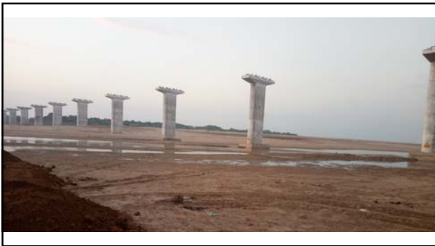
Fig. 159 Besides sand mining and water extraction, the mainstream Chambal is now becoming more accessible by road, from many crossings, such as this bridge under construction at Mandrayal-Sabargarh in the upstream NCS, crossing between Rajasthan & MP. At other localities upstream, bridges are planned or are under construction. Illegal sand removal increases when bridges and roads connect the river to roads. At present, four bridges are under construction in NCS.
