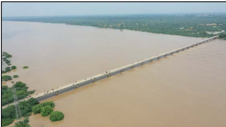
Fig.101 Aerial view of Sashon bridge shown in Fig. 102, showing the water level rise during peak rains, and the extensive flooding in the lower Chambal in August-September. River levels rise some 25-30 feet during the peak monsoon. During such periods, the gharial avoid the main channels, and prefer to use edges and back channels, where flow is minimal.
